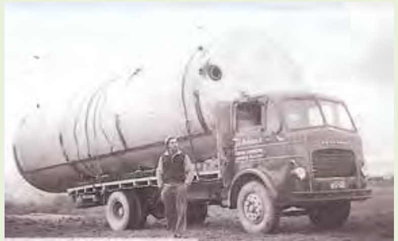
30' X 9' diesel fuel tank being delivered to the Lucerne Meal Factory from the rail head.
