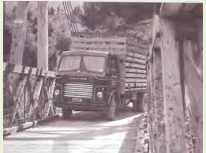
Negotiating the Lime Stone bridge Awatere Valley.
