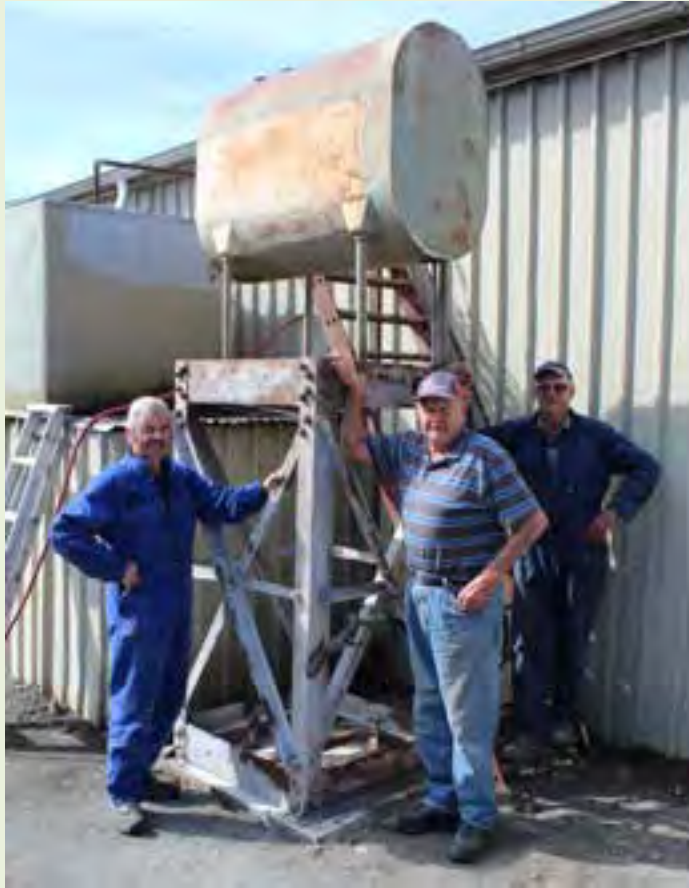
The diesel fuel tank outside the engine shed with the new concrete footing, steel support frame and the set of stairs to allow easy access to the fuel tank.
