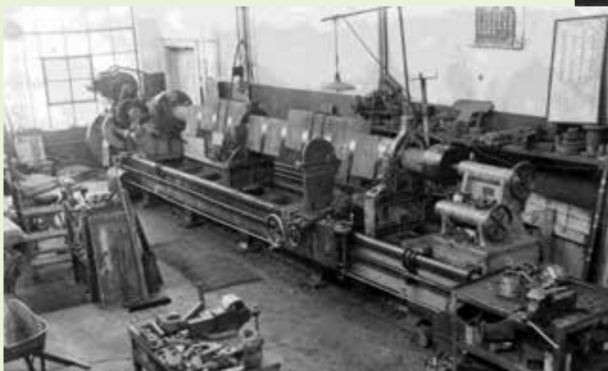
A crankshaft for a ten cylinder is set up and ready to be machined. The calendar on the wall above the lathe is June 1943
